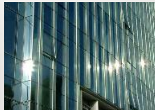
Centralized procurement of lighting roof shading coating
