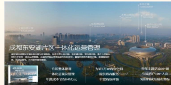
Chengdu Dong'an Lake Integrated Project
