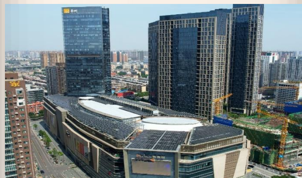
Zhengzhou MIXC rooftop photovoltaic
