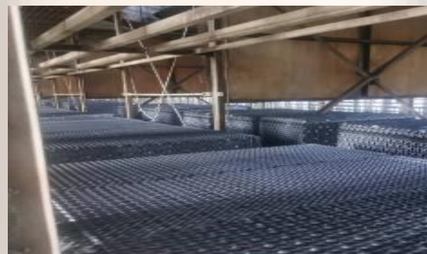
China Resources Tower air conditioning renovation
